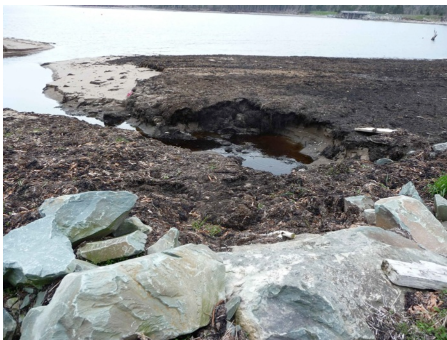
Figure 5 Downstream end of culvert buried by armour stone, and the temporary channel that was created by the spring freshet. Photograph by T. Bowron, 25/6/11.
