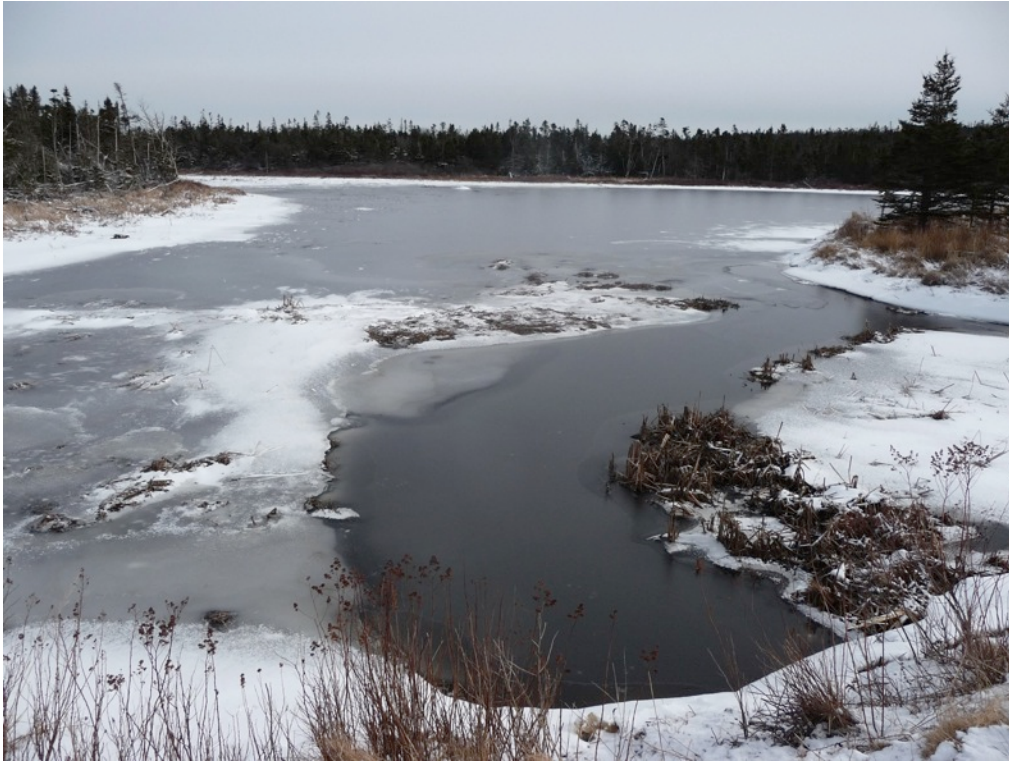
Figure 4 Upstream side of culvert and road.
